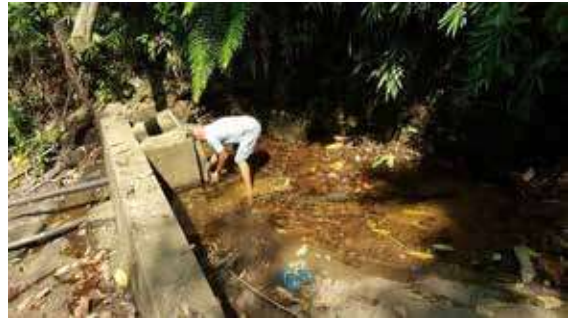
Figure 3 - Yatadollawaththa Water Supply
