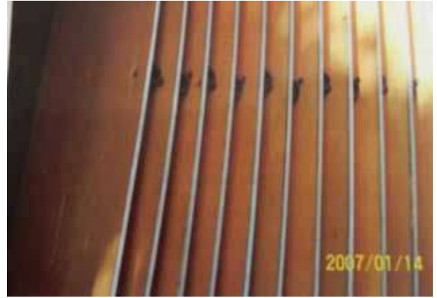
Figure 3 - Fixing details of plate settlers
