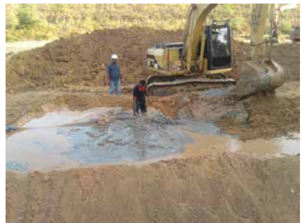
Figure 3 - Mixing of soil, cement and bentonite at mixing pad using excavator
