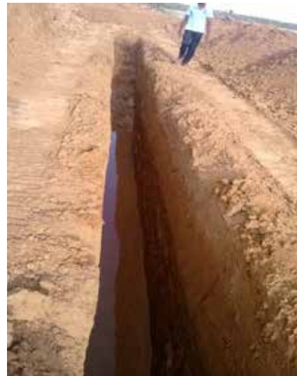
Figure 5 - Trench filled with bentonite
