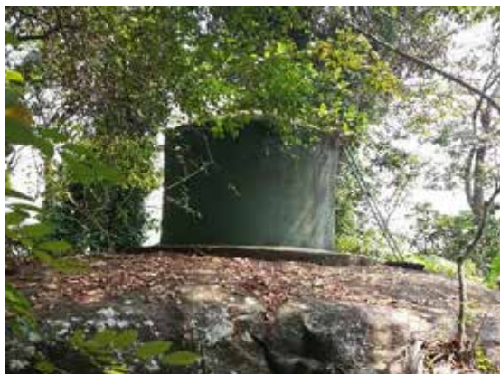
Figure 7 - Storage Tank, Welipenna
