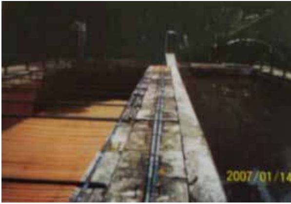
Figure 2 - Plate settler sedimentation tank after completion (2007)
