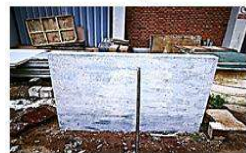
Figure 5 - Casted filler slab (a) and RC solid slab (b)
