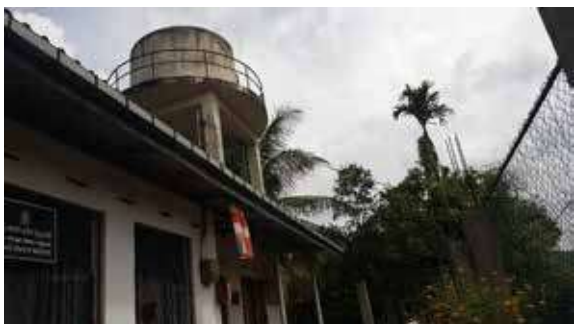
Figure 6 - Storage Tank, Kumbuka, East
