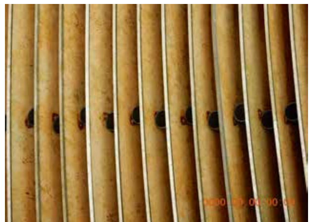
Figure 6 - Fixing details of plate settlers after 10 years
