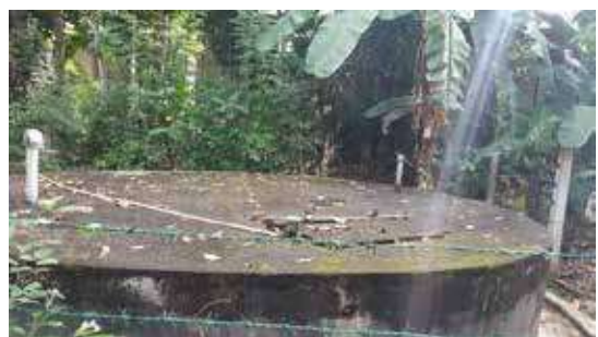
Figure 4 - Dug Well, Kumbuka West
